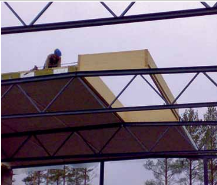
Ferdig montert karm
